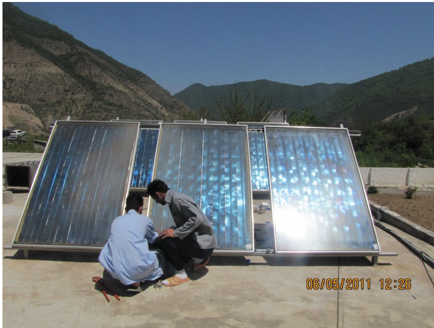
Personnel bathroom of Talavang North Company, Paran Farm, with a capacity of 1600 liters – Mazandaran
